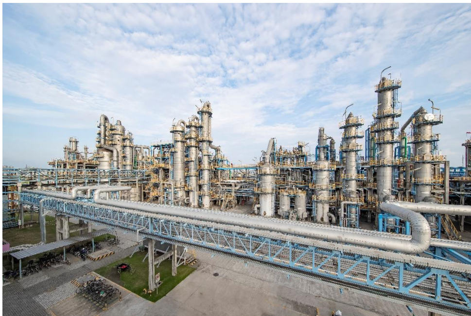
Röhm’s integrated methacrylate production facility in Shanghai.
